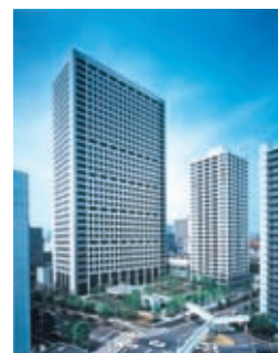
Granpark: NTT Group companies took the place of a key departing tenant, which has succeeded in reducing vacancy risk.
