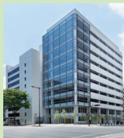
Urbannet Kotodai Building (Sendai-shi, Miyagi)
