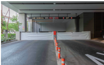
Flood protection sheets
