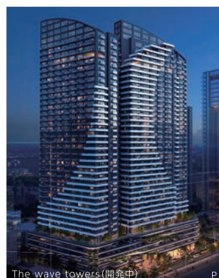
The wave towers (開発中)
